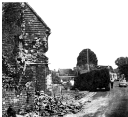
A common occurrence – a lorry has shed its load after hitting the corner of Bubblestone Farm only a few feet away from the main road.
